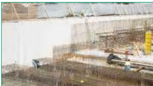
Steel reinforcement being placed in front of BENTOFIX®.
