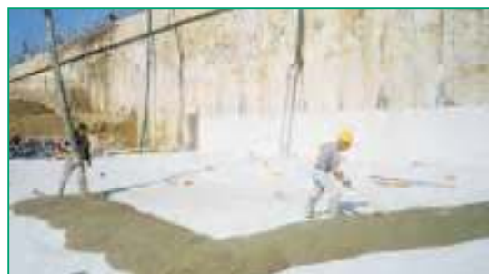
Pouring of concrete over BENTOFIX®.
