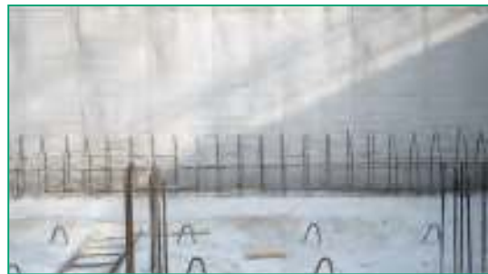
Vertical fixing of BENTOFIX® against a concrete face.
