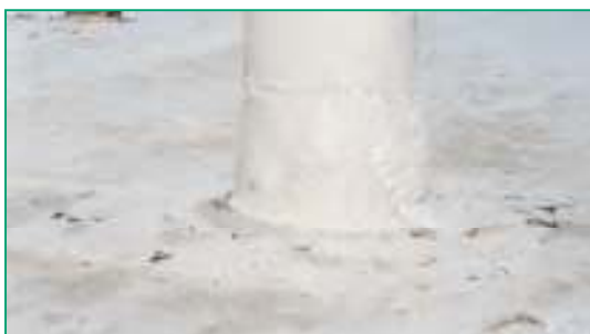
Sealed pipe penetration with BENTOFIX®.
