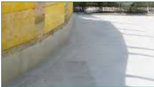
Vertical fixing of BENTOFIX®.
