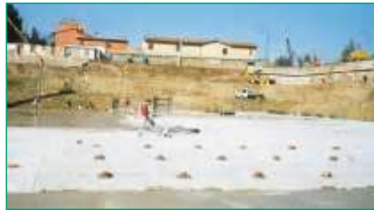
Unrolling of BENTOFIX® membrane on a base.
