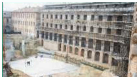
Waterproofing site with BENTOFIX®.
