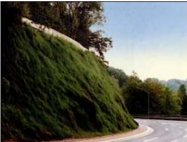
Steep slope after Hydroseeding
